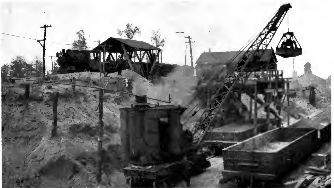
General view, showing one phase of York Sand & Gravel Company's operations.
